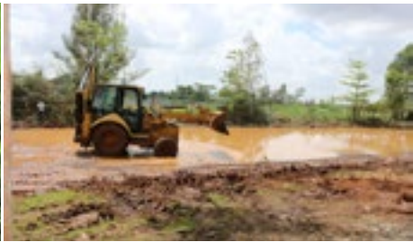
Ongoing excavation and reclamation in readiness to lay the foundation
